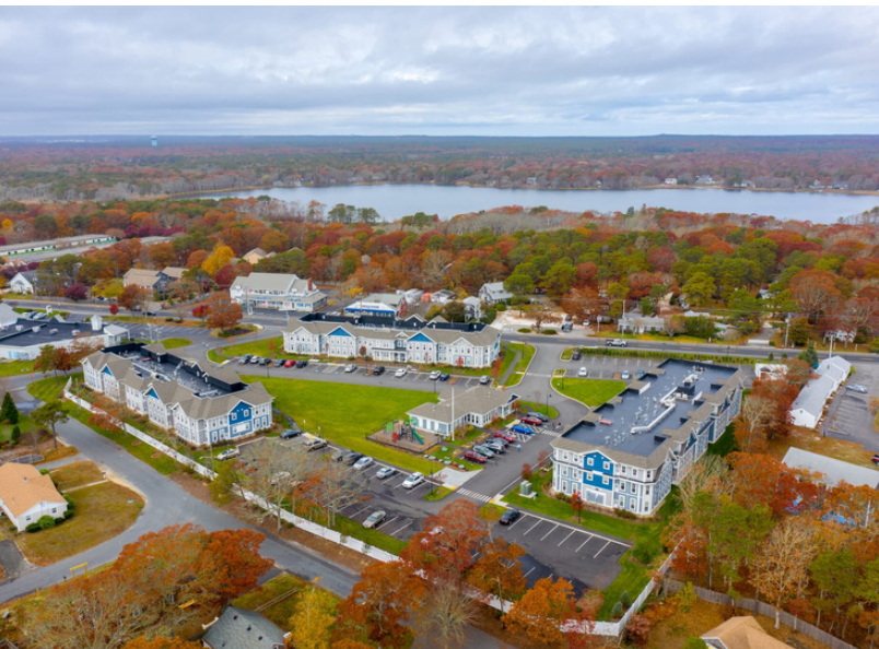
Yarmouth Commons – 69 affordable rental units made possible through Yarmouth's Motel Redevelopment Program.
